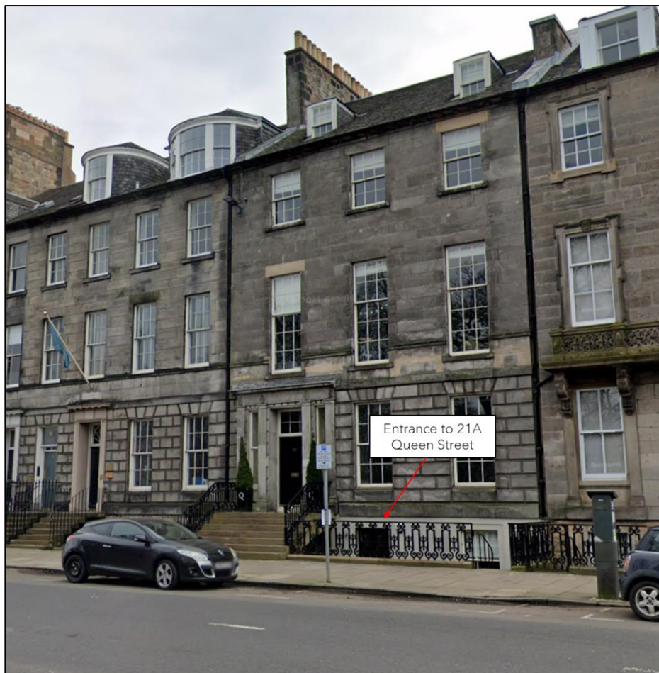
Figure 1: Entrance to 21A Queen Street, and neighbouring uses
